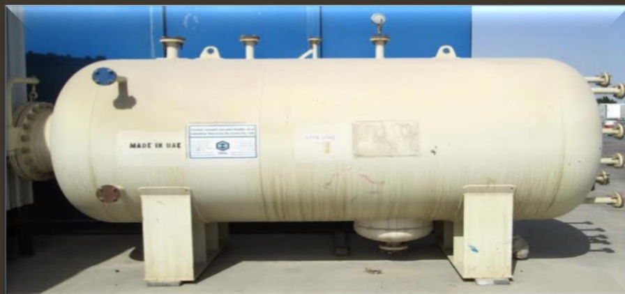
AIR RECEIVER: CAPACITY : 10000 , 5000, 3000 LTS.
